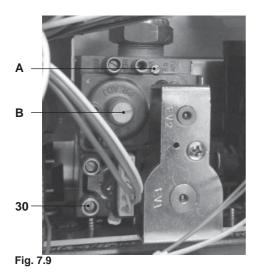
If it does not comply with the required pressure check the gas supply line and governor for faults and/or correct adjustment.
